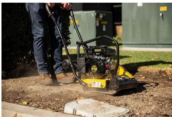
Figure 59: A compactor densifies the sand.
