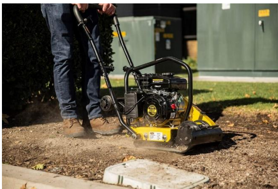
Figure 59: A compactor densifies the sand.
